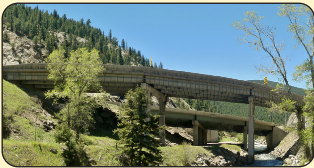
Image 20. I-70 over US 6 and Clear Creek in Clear Creek County (F-15-BL)
