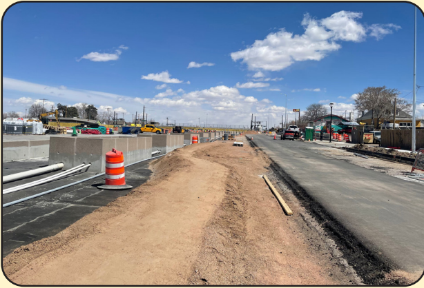
Image 13. Construction on 46th Ave.
