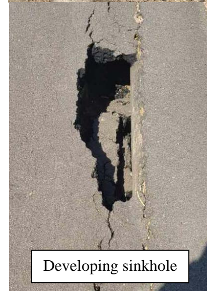
Voids under slope paving
