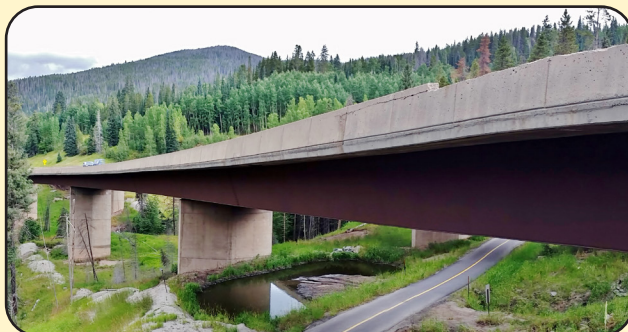
Image 18. I-70 EB over Polk Creek in Eagle County (F-12-AS)
