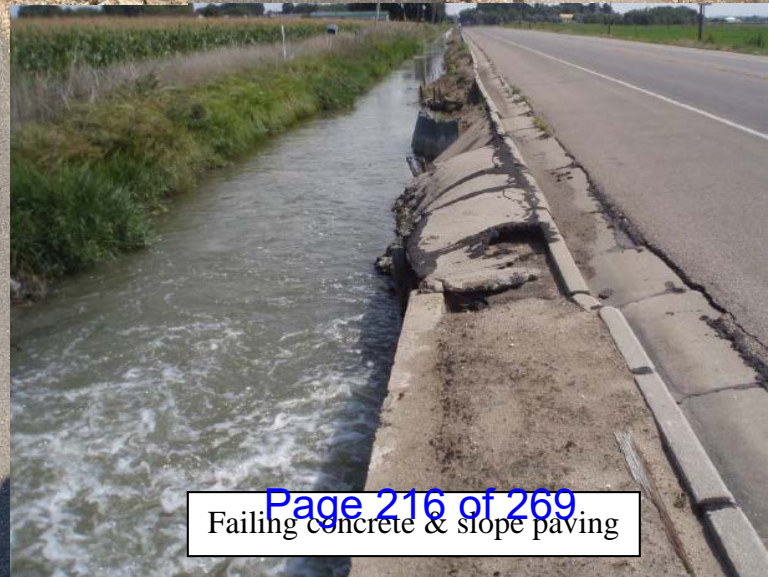
Broken & Settled Curb line
